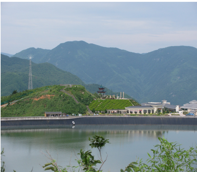
Fig. 1 Observational site – upper reservoir of the Pumped Storage Power Station at Tianhuangping, China
