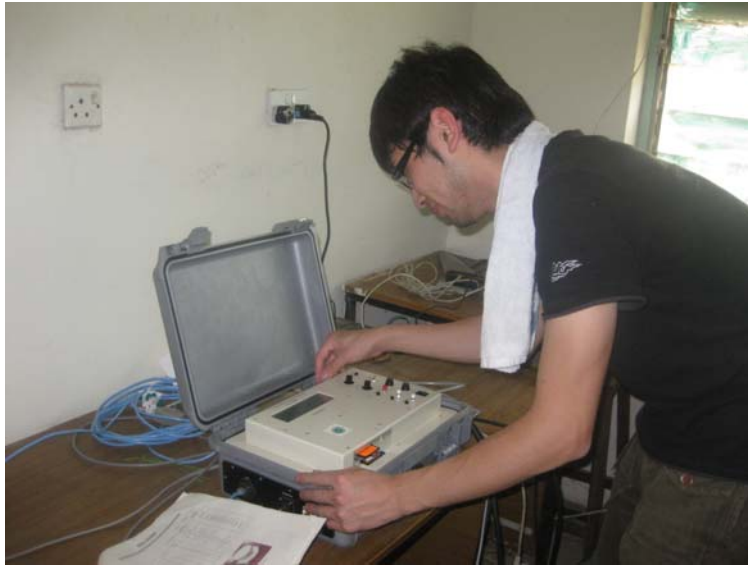
Fig. 4: The Data logging and Transmitting Unit of the Magnetometer
