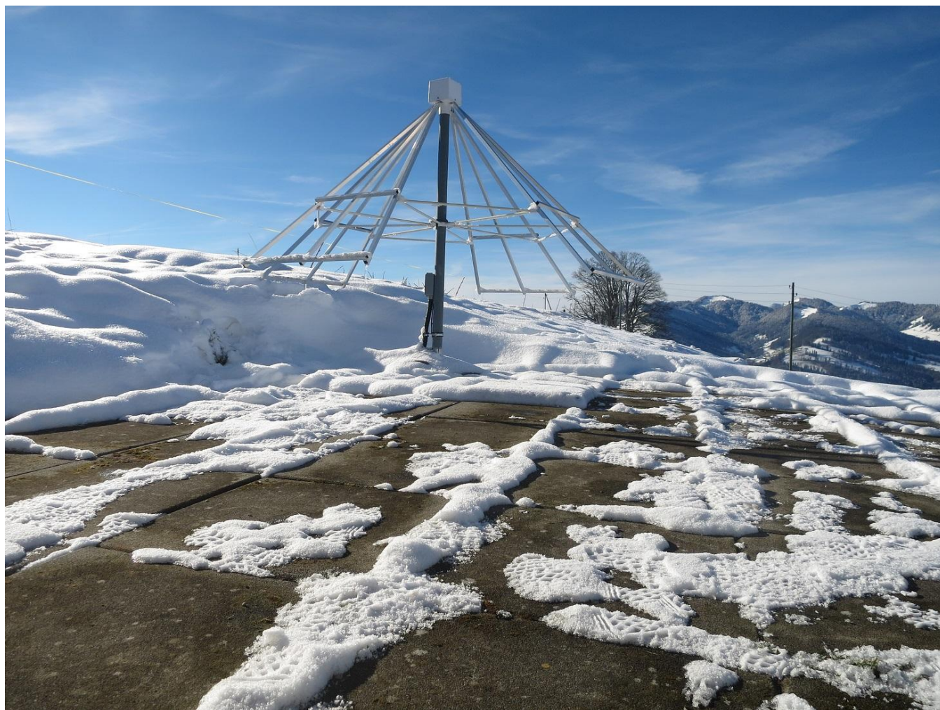
Fig. 1: LWA installed at observatory "Scherrer" in Heiterswil, Switzerland.
