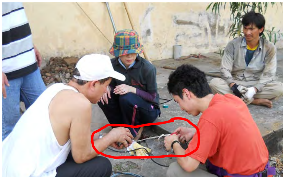
Pulling sensor cable through buried tube.
