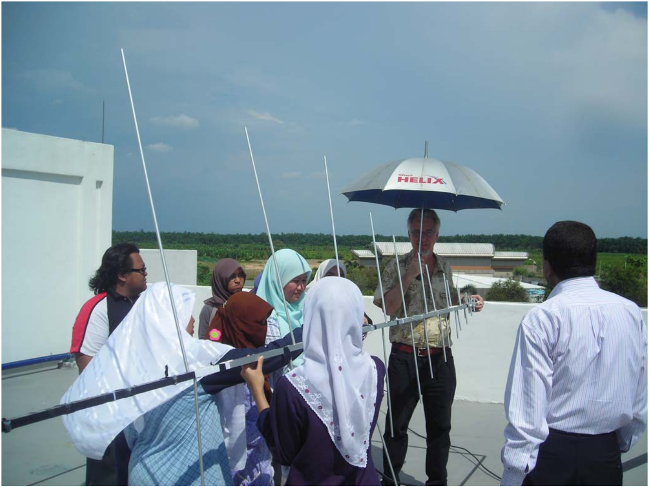
Fig. 3: Logarithmic-periodic antenna built at ANGKASA covering about 100 MHz – 900 MHz. Students install the coaxial cable to one of the booms of the antenna. Outside temperature was +37° C.
