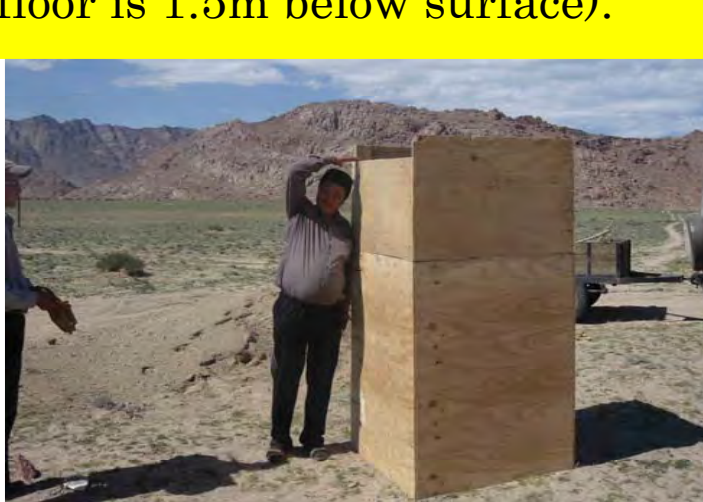
Construction of sensor house (floor is 1.5m below surface).
