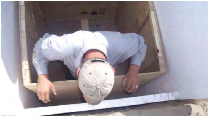
Construction of sensor house (floor is 1.5m below surface).
