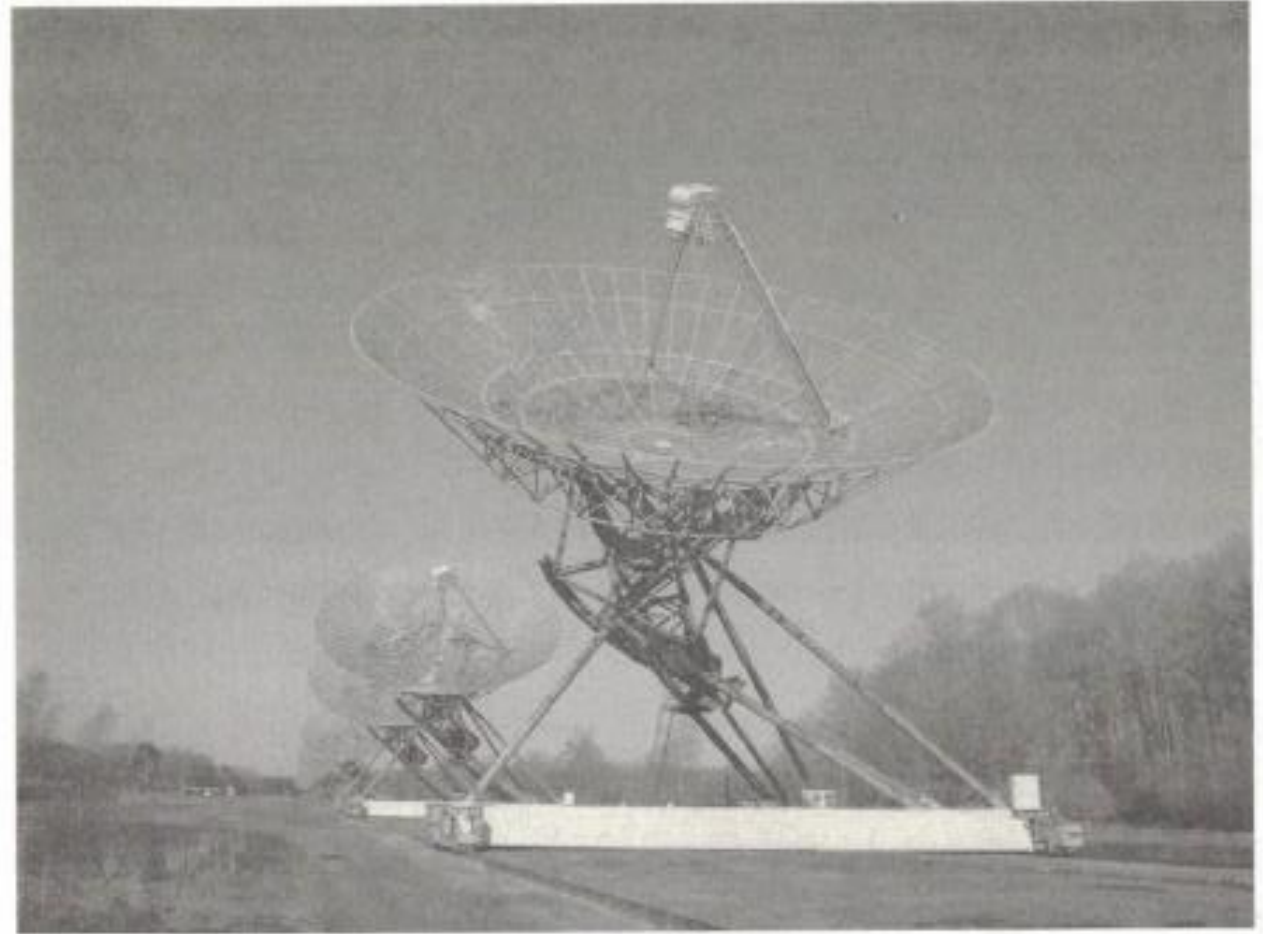
FIGURE 56 The Westerbork Synthesis Radio Telescope (WSRT). Each of the 14 parabolic reflectors is 25 metres in diameter. © Chris Sciacca, IBM Research.
