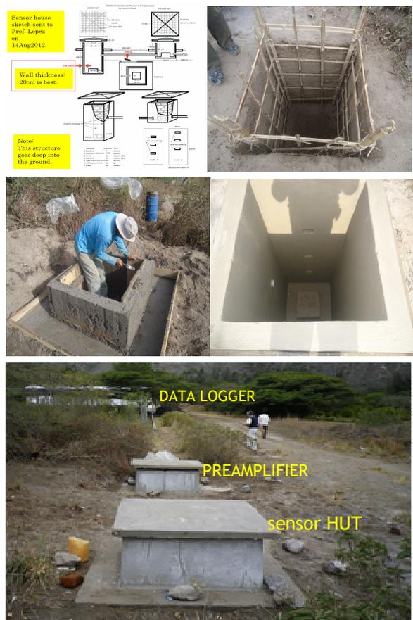
Figure 3: Houses for sensor HUT and preamplifier construction
